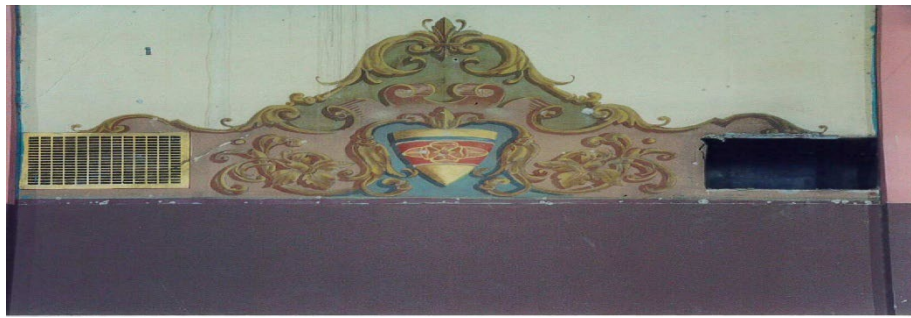
Figure 16: Original scrollwork and cooling system ducts on the interior of the theater, taken in 1998 as part of the restoration.
