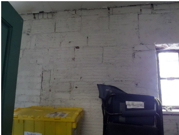
Figure 8: Photo of the building's interior, documenting use of hollow clay tile and brick in construction.
