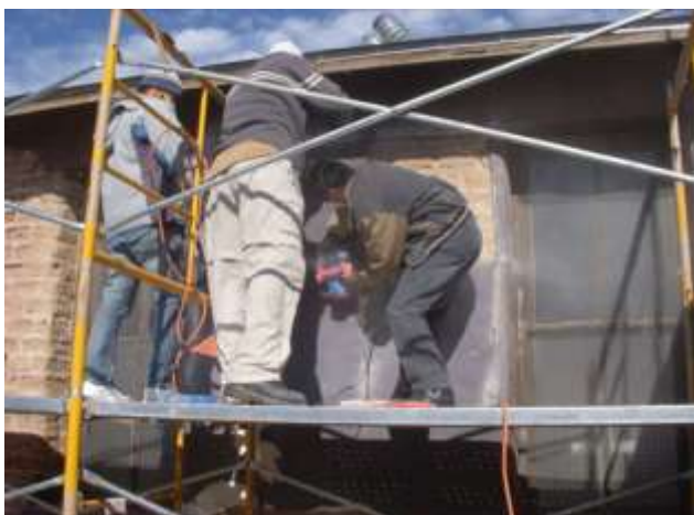
Figure 24: February 2010 removal of cement stucco south side of Chapel. (Courtesy of Faith Hutson).
