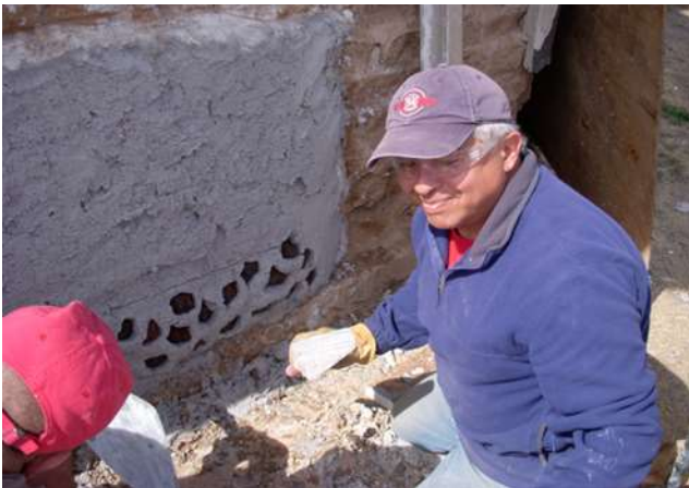
Figure 28: Application of lime plaster and rajuelas to the apse wall by David Chavez, Spring 2010. (Courtesy of Faith Hutson).
