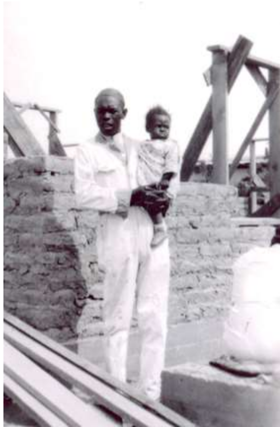
Figure 12: Henry Fielder with one of his sons, either Alfred or Cleo, at the home construction site, 642 E. Court Street, date unknown. (Courtesy of Clarence Fielder).
