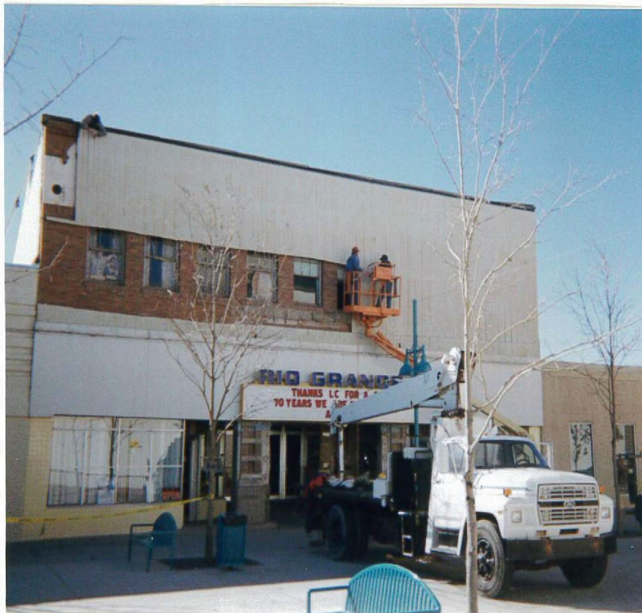
Figure 13: Photo from 1998, during removal of the false front.
