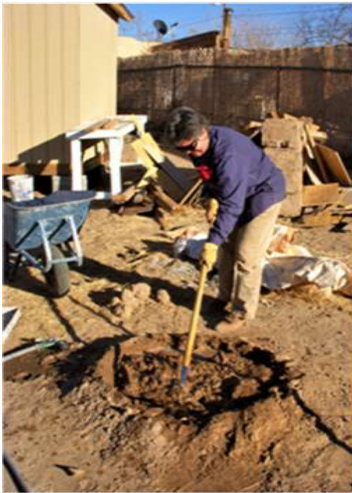
Figure 38: Stacia Fine mixing a volcano of mud mortar, 2011. (Courtesy of Faith Hutson).
