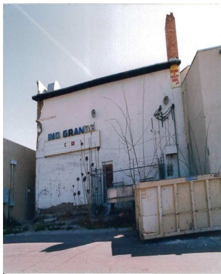
Figure 17: Rear of the theater during the 1998 restoration.
