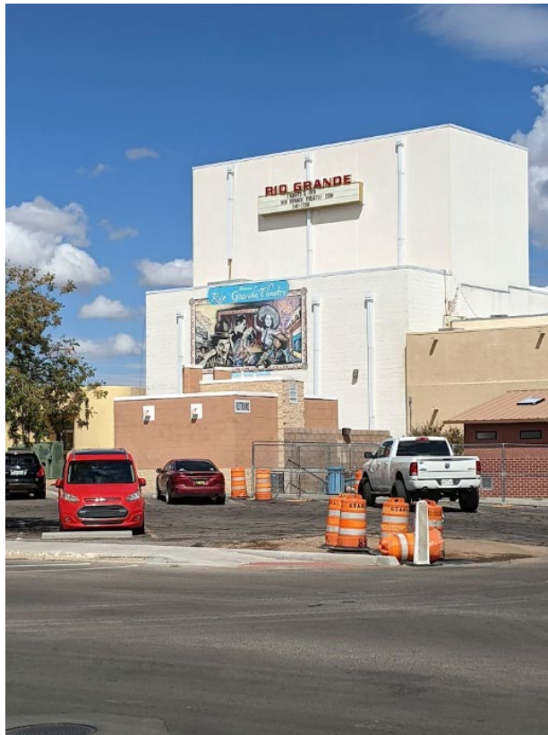
Figure 3: View of rear of building, facing northeast, capturing an old marquee, still in use. Photo includes non-historical mural.
