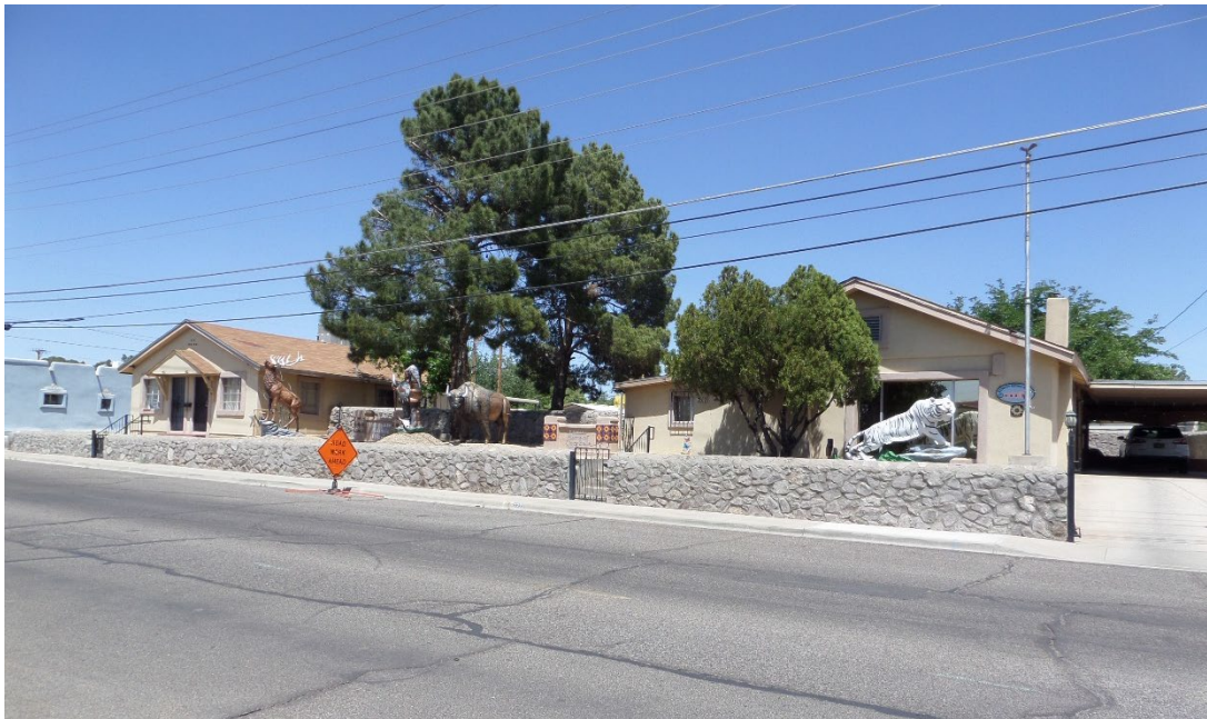
Figure 1: The two buildings that make up the Clara Belle Williams property from Mesquite Street; the Williams house, 722 N. Mesquite, is at the left, with the duplex at 734 N. Mesquite on the right.
