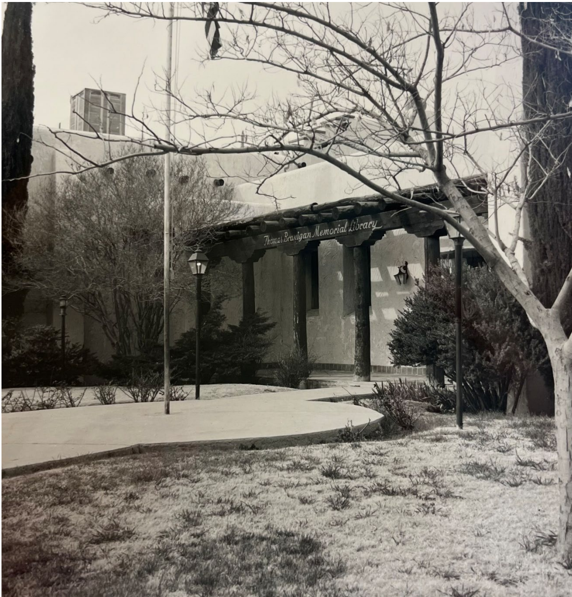
Figure 12: Photo of the building, dating to the 1960s. NMSU Archives, Rio Grande Historical Collections.
