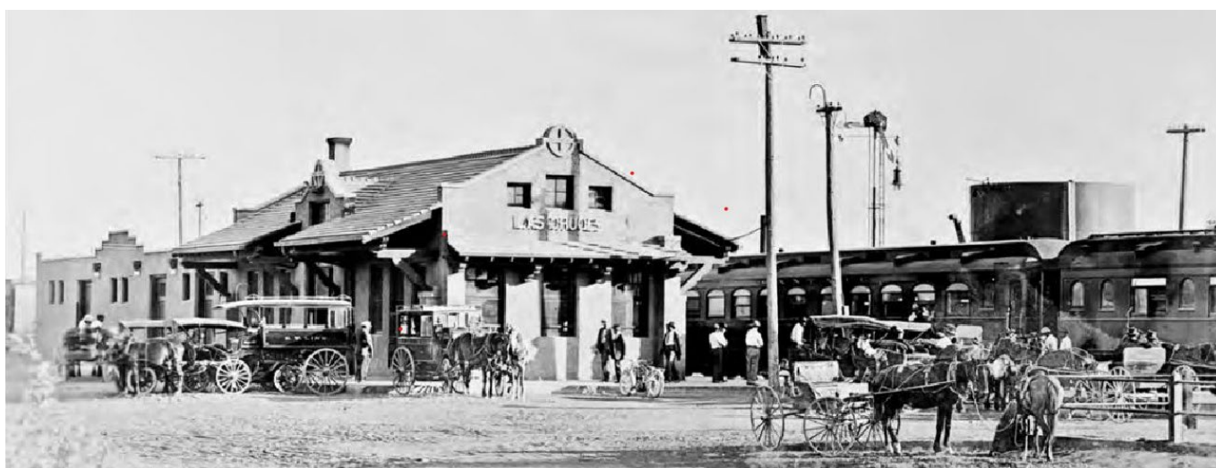
Figure 14: The depot from the northeast, circa 1910 (courtesy of NMSU archives, Rio Grande Historical Collections).
