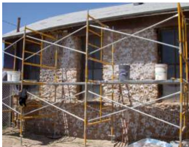
Figure 25: Application of rajuelas on the south side wall April 2010. (Courtesy of Faith Hutson).
