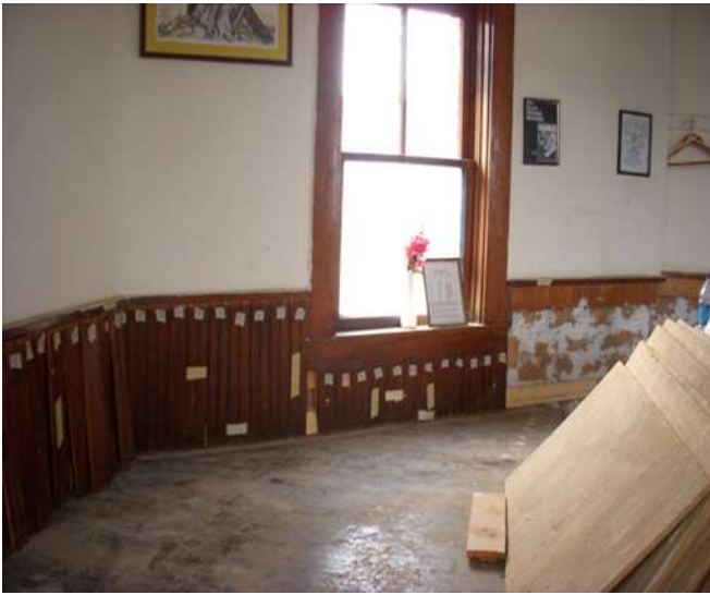
Figure 26: Inside wall repair April 2010. (Courtesy of Faith Hutson).
