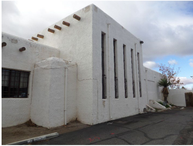
Figure 3: Rear of the building, facing south.
