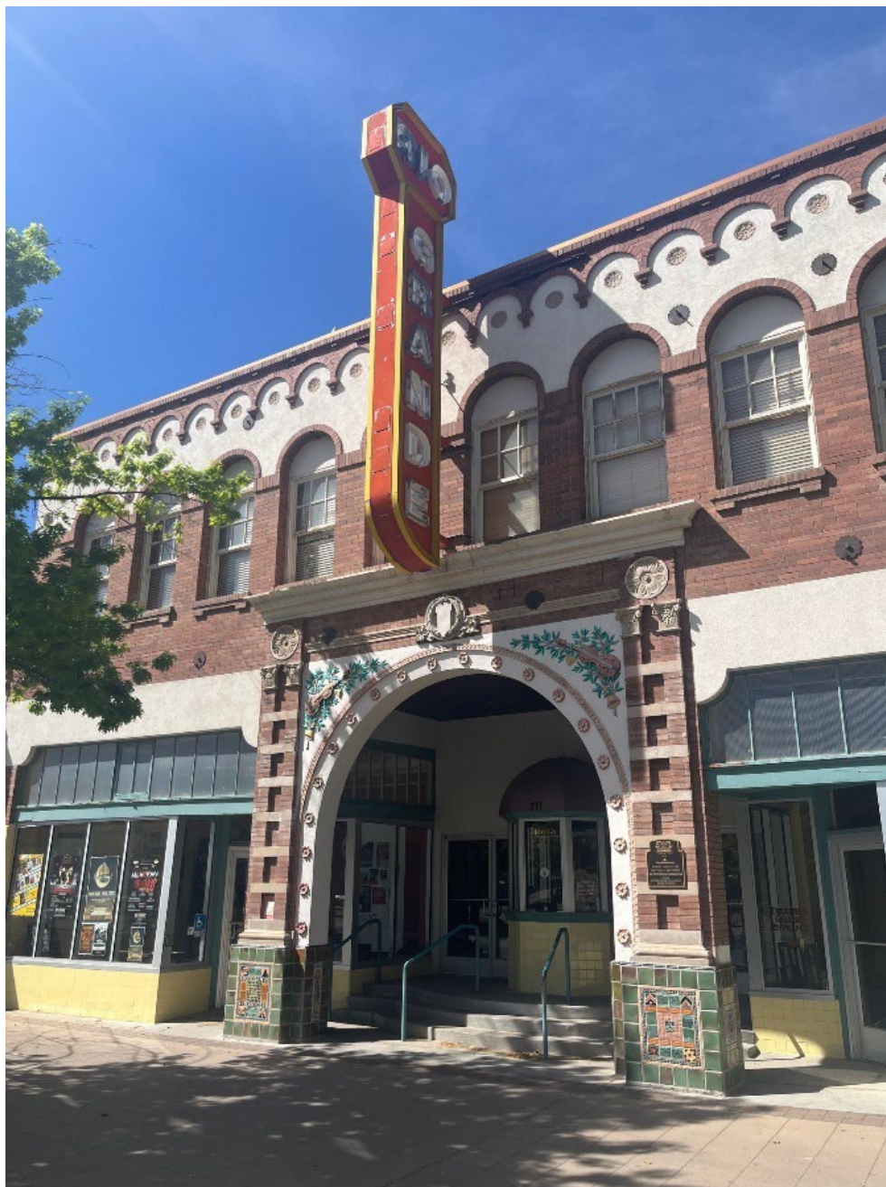
Figure 1: Front of building and marquee tower, facing southwest.
