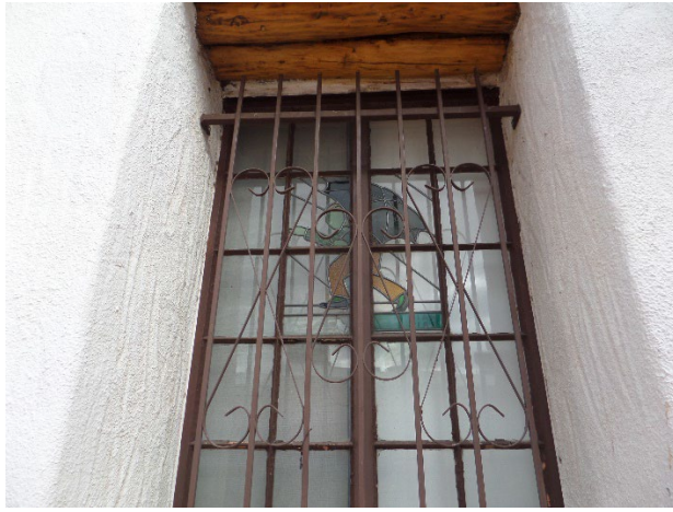
Figure 6: Stained glass on the south side of the building.
