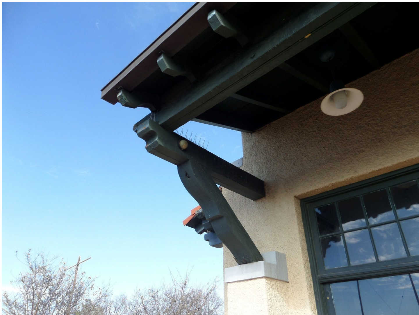
Figure 6: Ornately carved wooden brackets support the building's extended roof eave, photographed on the west side of the building.
