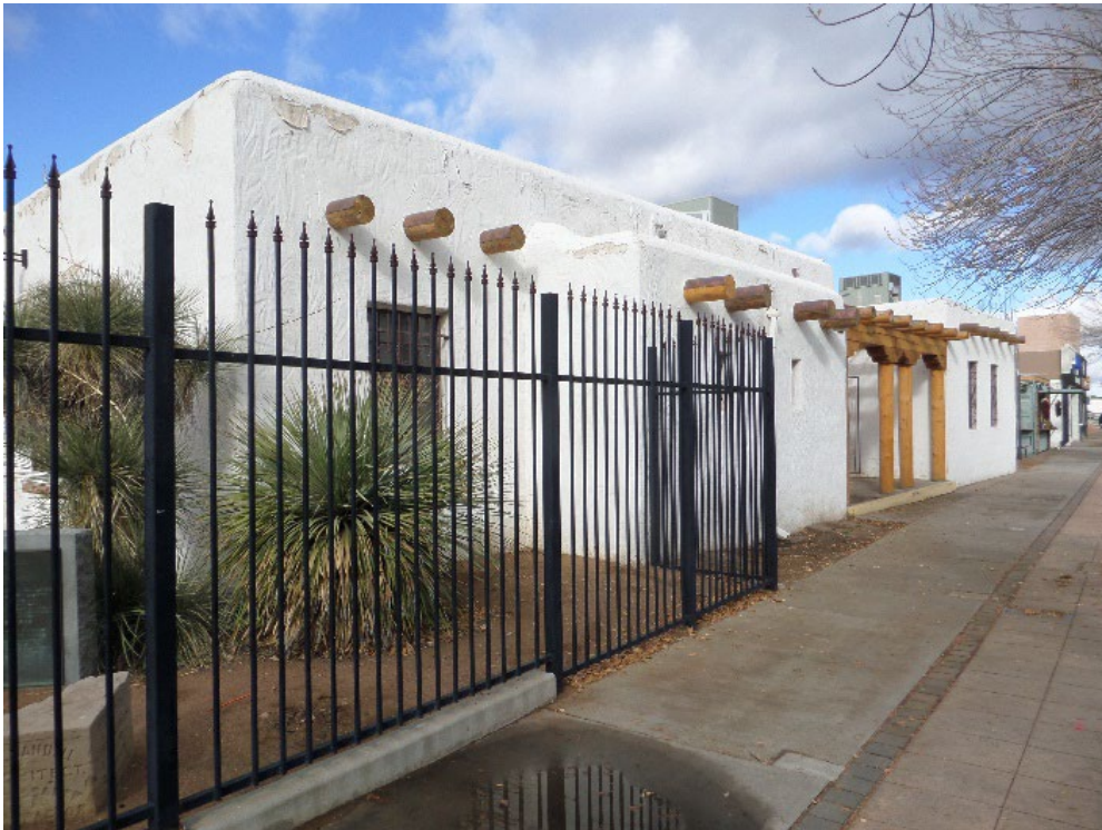
Figure 2: Photo from the sidewalk on Main Street, looking northwest at the east façade of the building.
