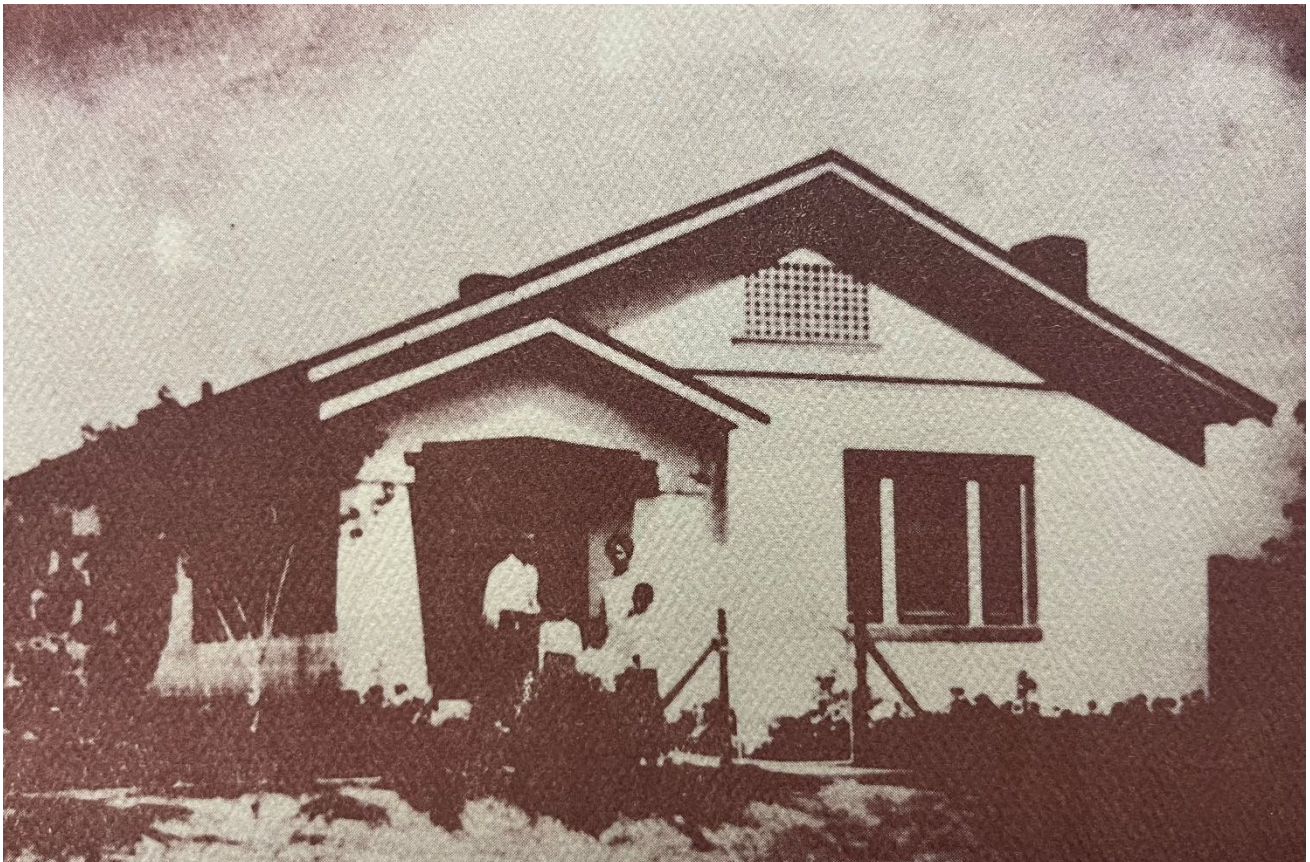
Figure 5: Historic photo of the Williams family in front of their house at 722 N. Mesquite Street (retrieved from “The Las Cruces Historic Buildings Survey”).
