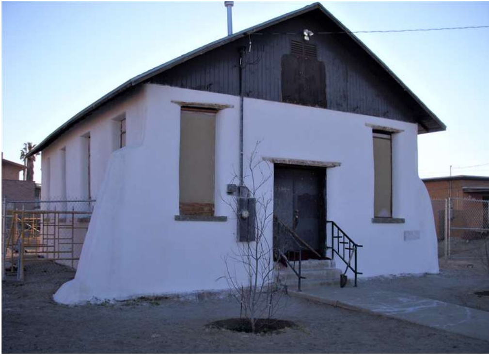
Figure 47: Church with final coat of line plaster called the sugar coat. Note the completed windows cover with paper, 2013. (Courtesy of Faith Hutson).
