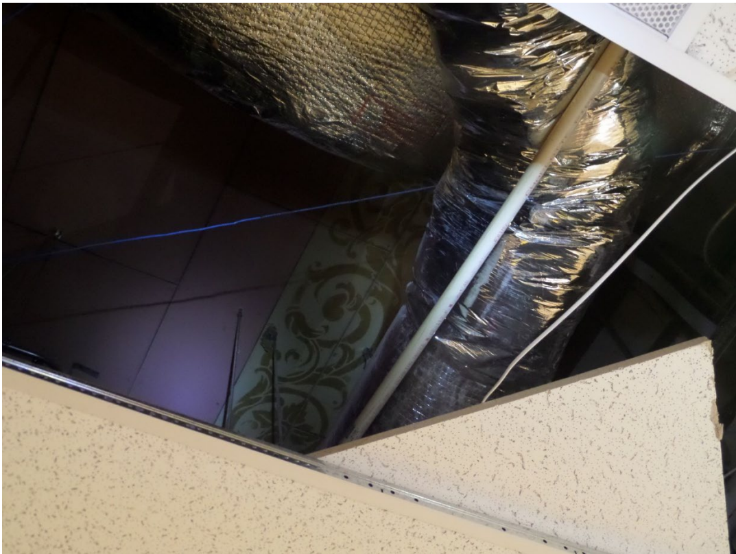
Figure 5: Rinceau motifs on the original ceiling of the balcony, visible behind the drop-ceiling of the second-floor offices.
