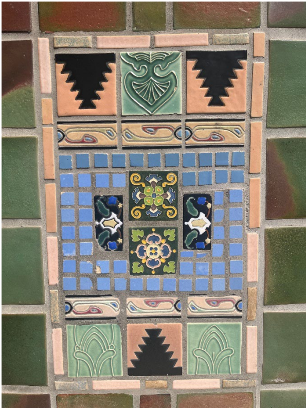
Figure 10: Replicated tiles on the theater exterior.
