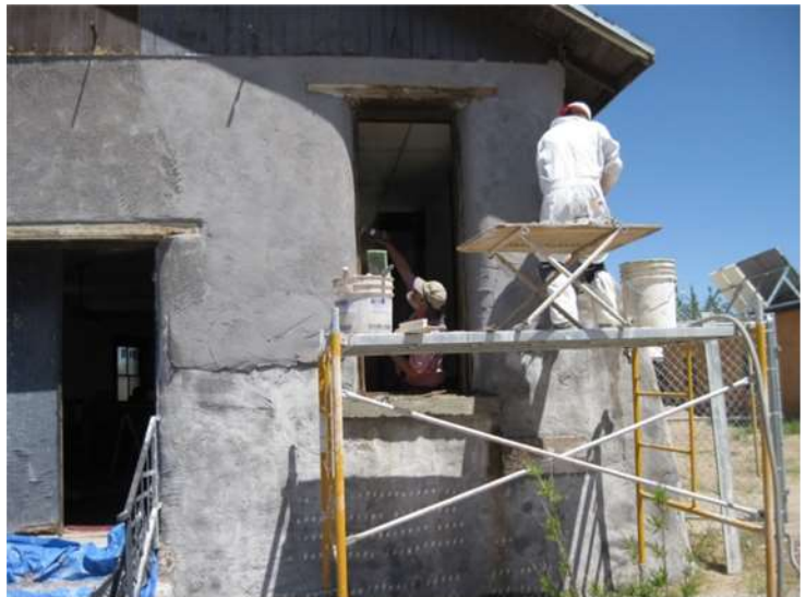
Figure 46: Lime Plaster application to front façade. John Hyndman in the window opening, Larry Limon on the scaffolding, 2013. (Courtesy of Faith Hutson).
