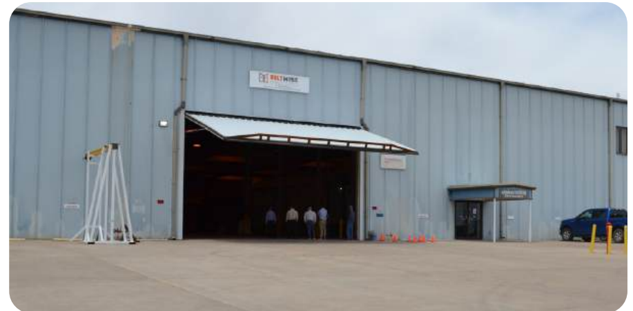
Figure 2.10: Industrial Building, BiltWise
