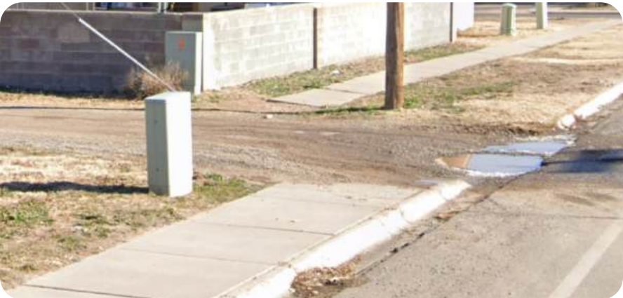
Figure 6.13: Gap in Accessible Route on E. Berrendo Road east of Main Street
