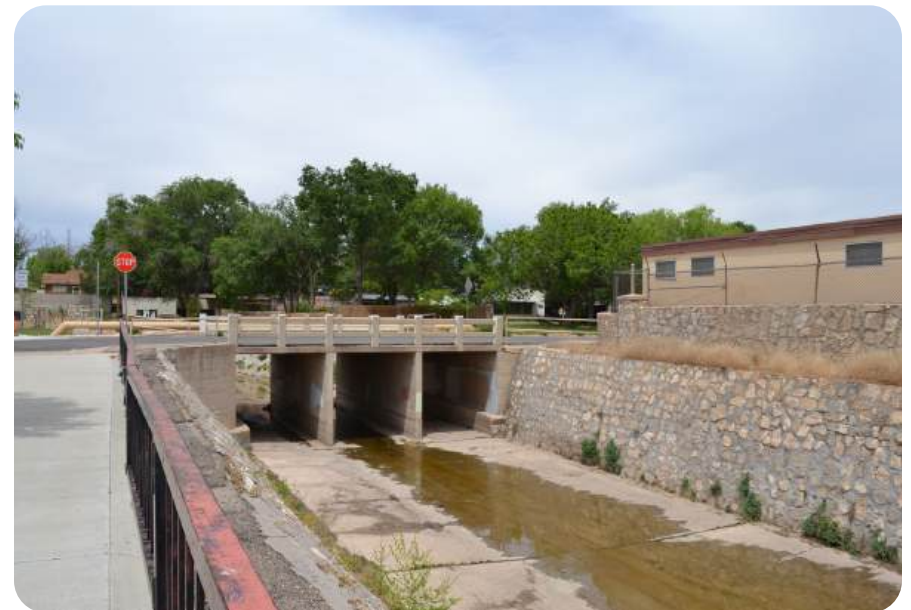
Figure 8.1: Bridge over the Spring River
