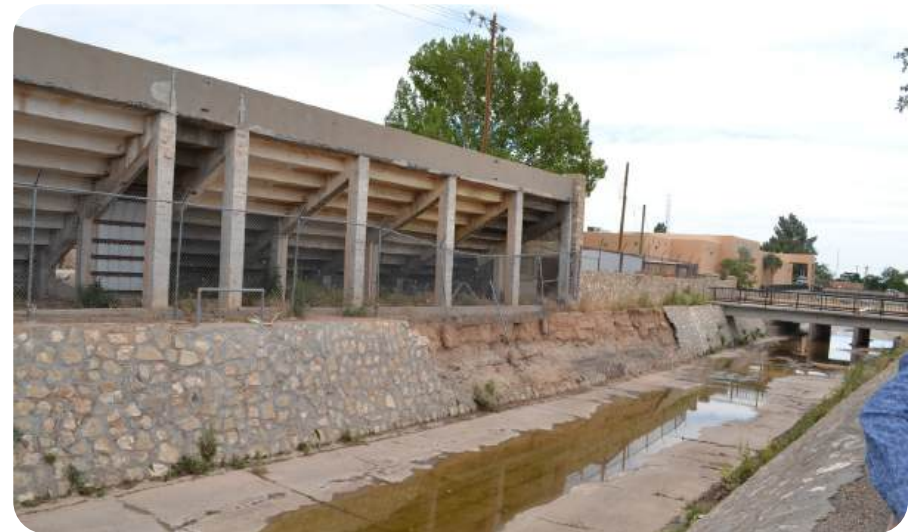
Figure 6.22 (A,B): Shows significant impervious surfaces throughout the city with very little on-site stormwater retention
