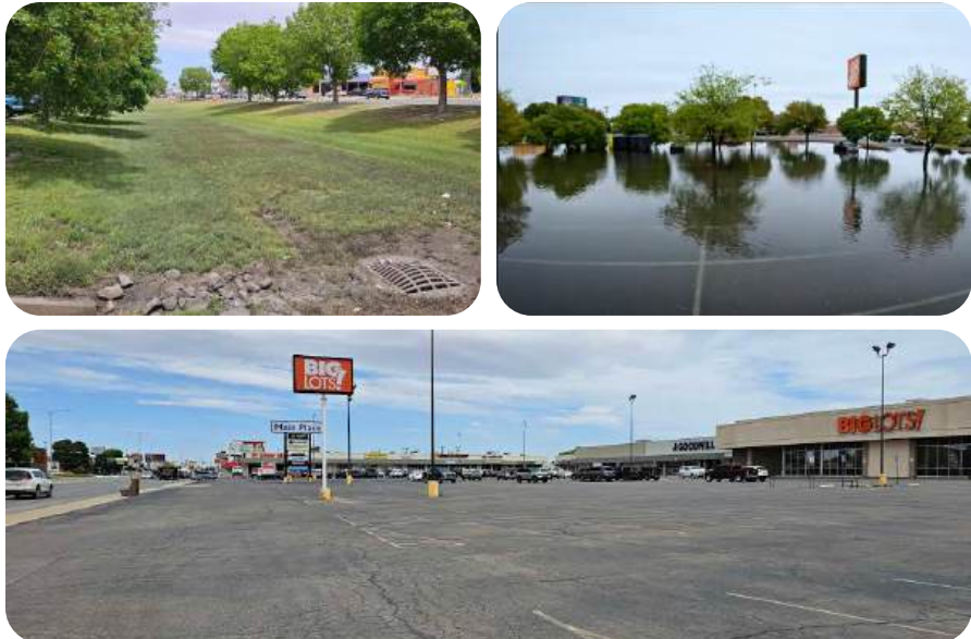
Figure 6.5 (A,B,C): Show On-site Stormwater retention at Home Depot Parking Lot on Main Street; Home Depot On-site pond after storm 2024; & Retail center on Main Street with significant area of impervious surfaces and no on-site stormwater retention.
