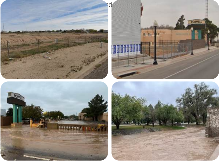
Figure 6.7 (A,B,C,D): Shows Existing Stormwater retention Basin at S. Cahoon Avenue and E. Buena Vista Street; Area Inlet on Main St. Near Spring River Crossing; Spring River crossing at Main Street & Spring River through Cahoon Park inundated during Storm 2024.
