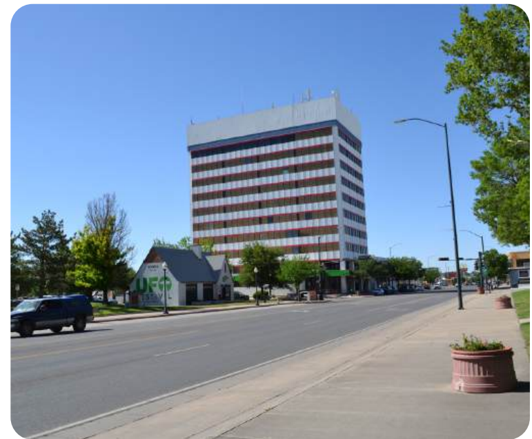
Figure 2.8: Roswell Sun West Centre Building
