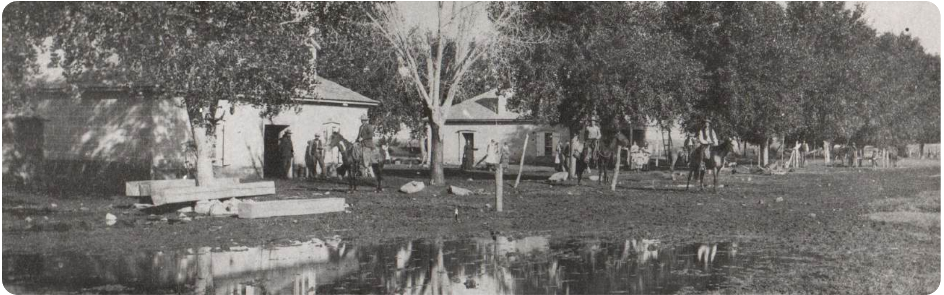
Figure 3.1: Picture shows the first two structures in Roswell according to the Roswell Historical Society. Shelter and housing has always been important to Roswell's growth. And it will continue to be a vital focus for its future.
