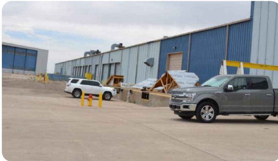
Figure 2.11: Industrial Building, BiltWise
