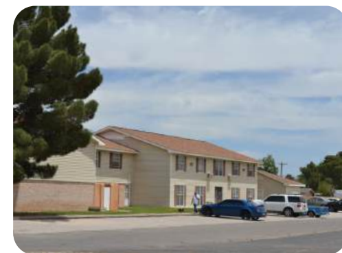
Figure 2.5 (A,B,C): Apartments and Duplexes in Roswell
