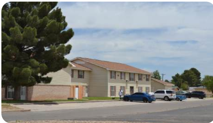
Figure 3.7: Residential Multi-Family Building
