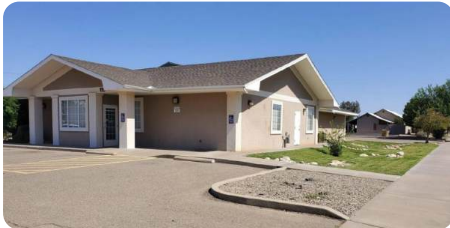
Figure 2.9: Roswell Mixed-Use Office Building
