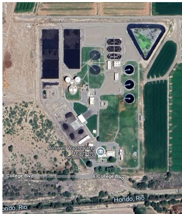
Figure 4 City Wastewater Treatment Plan
